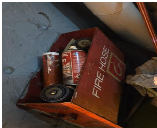
Fire hose box stowed with spares and tools
