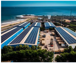
Construction of EXIM Godown Rs 43.91 Cr Tgt. Comp.: 30 th Sep'26
