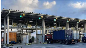
Gate Automation Rs 11 Cr
