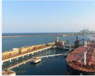
Augmentation of Fire fighting system Rs 43 Cr Tgt. Comp.: 31st Dec. 2026
