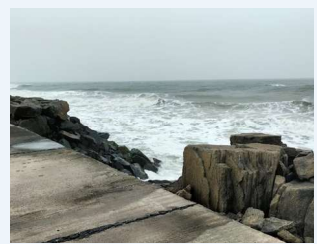
Strengthening of Revetment Rs 33.28 Cr Tgt. Comp.: 30th Mar'27
