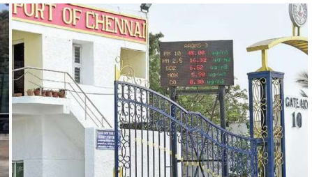
Continuous Air Quality Monitoring System
